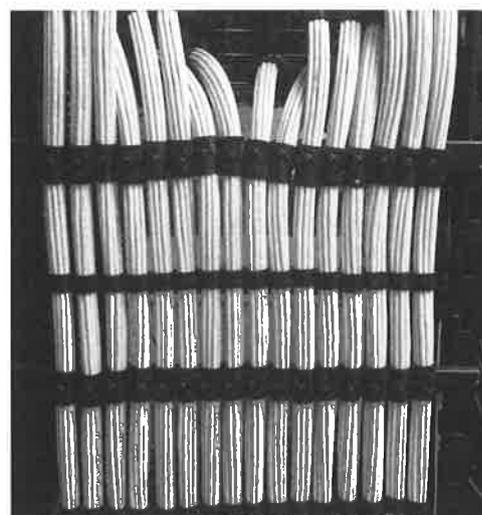
Figure 31: Soutagement de traction
